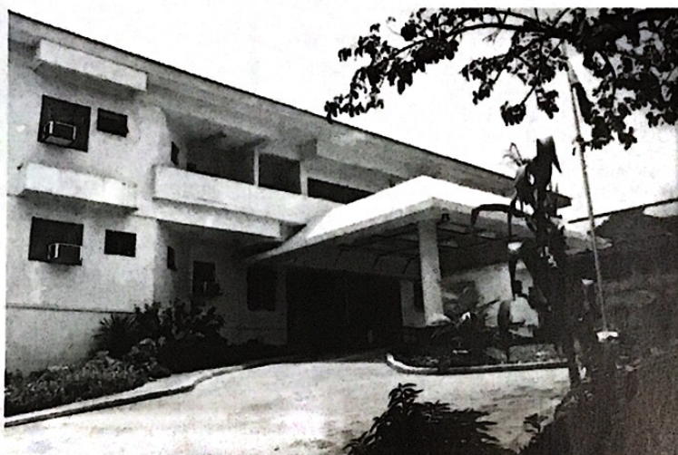
The 3rd floor of the CD building was completed in mid 2004.
